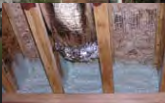
Foundation to deck closed cell foam sealing
