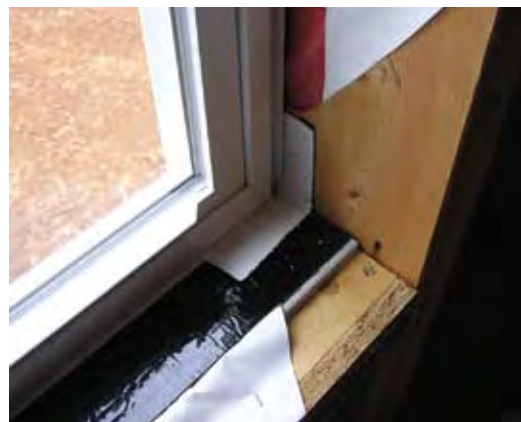
Sloped window sill flashing detail
